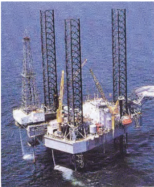
Offshore oil field using Cr bearing OCTG
